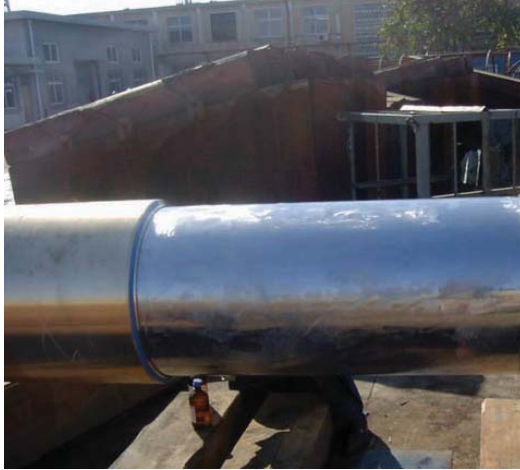
Shaft between liners is cleaned and prepared for shaft coating
