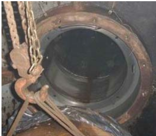
Inspect FWD and Aft stern tube
