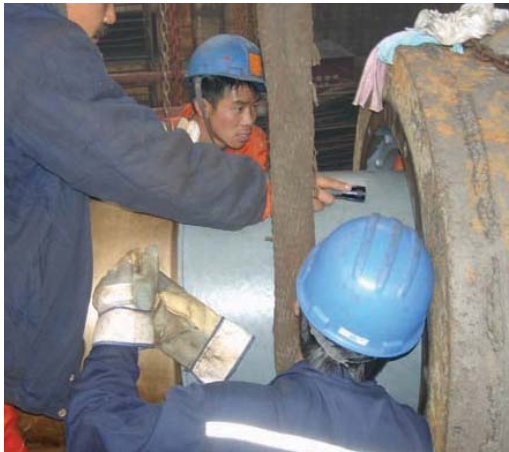
Shaft is fitted back into stern tube
