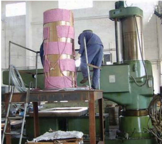
Liners are heated and shrunk fit to the shaft
