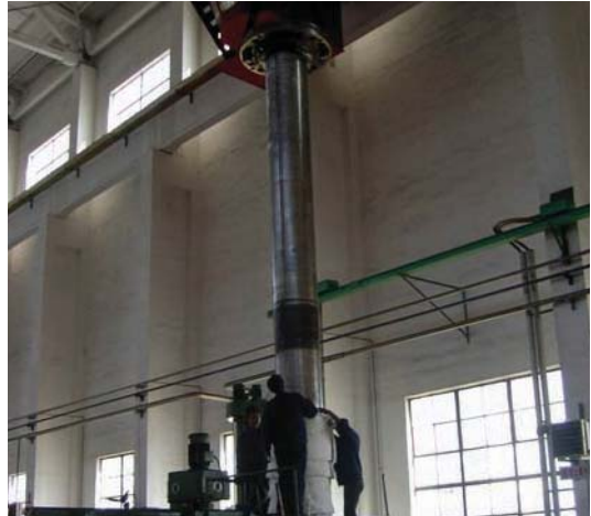
Shaft liner installation can be done horizontally or vertically
